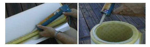
3. Place a bead of construction adhesive around the end of the pipe wrap. As with the seam make sure that there are no gaps. Place the end cap in place and insure that a good seal is obtained.
